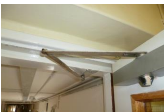
Overhead self-closer (image courtesy of Golden Thread Fire Delay)
